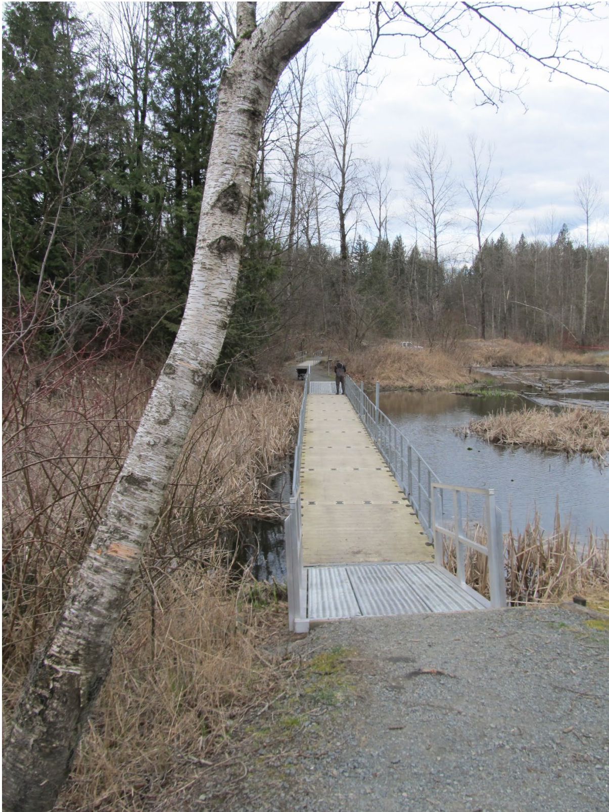
Photo 1: Segment 2 with ramp looking northwest
