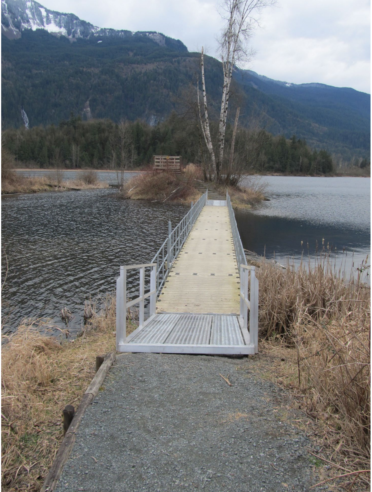
Photo 2: Segment 3 with ramp looking south
